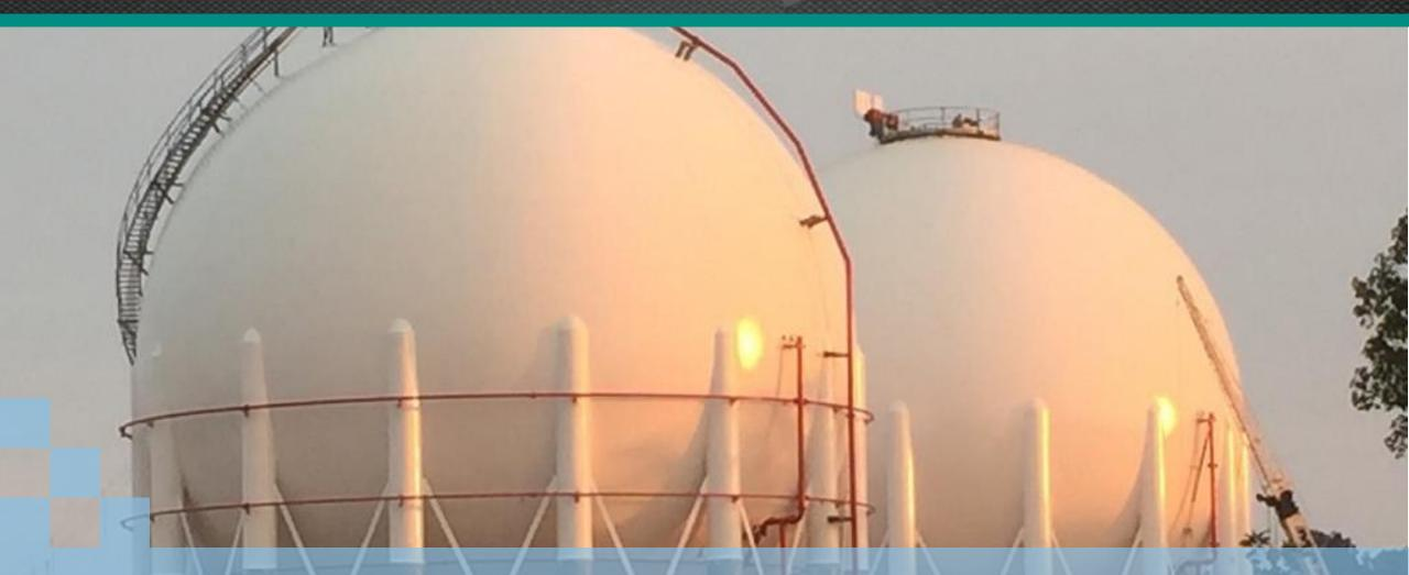
✓ Storage and distribution of liquefied petroleum gas (LP Gas) with a capacity of 40,000 nominal barrels.
