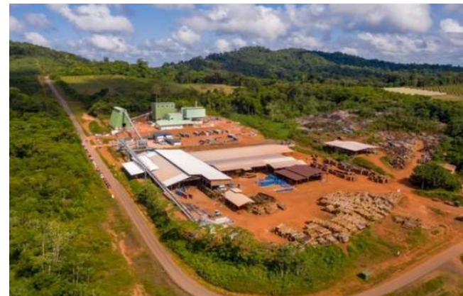
5.1 MW Biomass plant French Guyana (2021)
