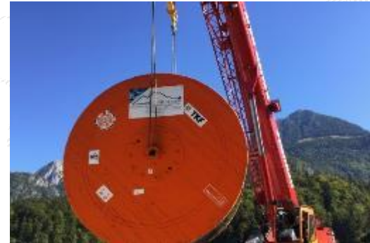
Subsea cable connection Germany 2015, Germany Client: Wiking Kabel
