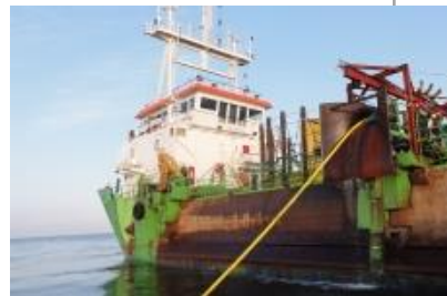
2006 First offshore power cable project
