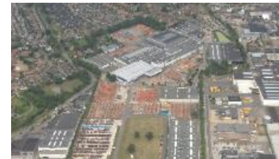
2010 Integration production locations All under one roof, location Haaksbergen
