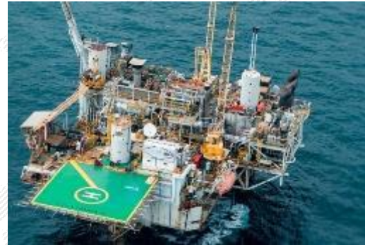
Replacement subsea cable Perenco 2016, Gabon Client: Perenco
