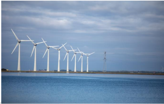
Inter-array cable offshore wind park Windplan Blauw – 33kV 2022, Netherlands Client: Ballast Nedam
