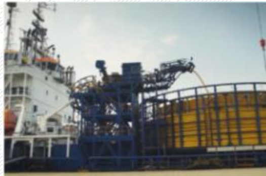
Inter-array cable offshore wind park Albatros – 33kV 2018, Germany Client: EnBW
