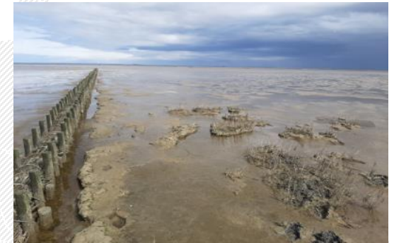
Subsea cable connection Holwerd– Ameland connection –33kV 2021, Netherlands Client: Liander
