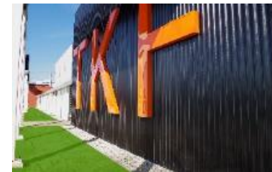
Subsea production plant Opening state-of-the-art subsea production plant Lochem (NL)
