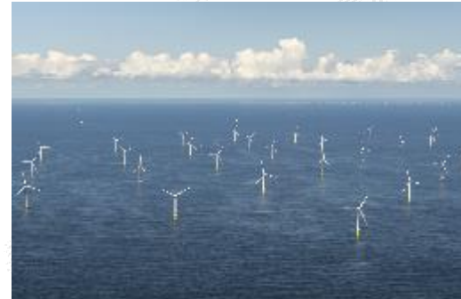
Inter-array cable offshore wind park Hollandse Kust Noord – 66kV 2021, Netherlands Client: Van Oord
