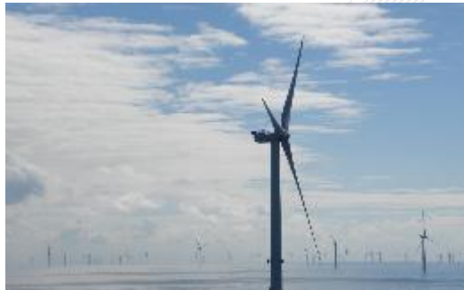
Inter-array cable offshore wind park Hollandse Kust Zuid – 66kV 2020, Netherlands Client: Vattenfall
