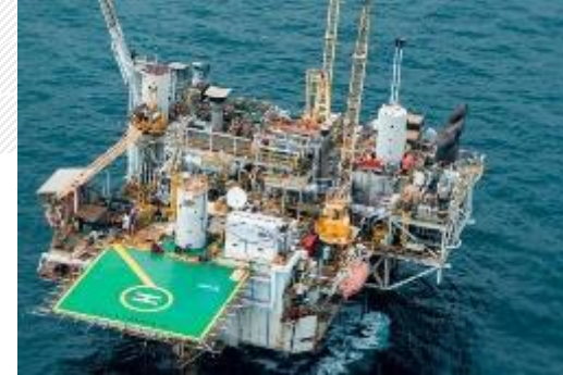
Replacement subsea cable Perenco 2015, Gabon Client: Perenco
