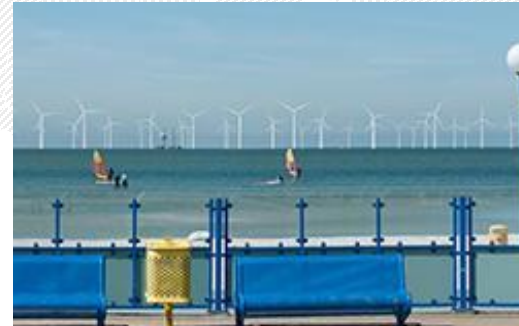
Subsea cable connection Windpark Fryslân – 33kV 2020, The Netherlands Client: Van Oord
