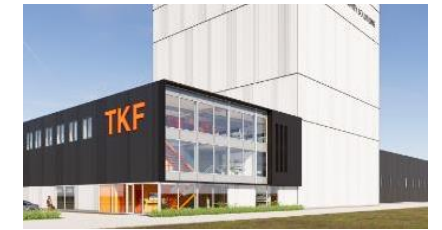
Expected 2023 opening factory Opening production plant ready for 132 kV in Eemshaven
